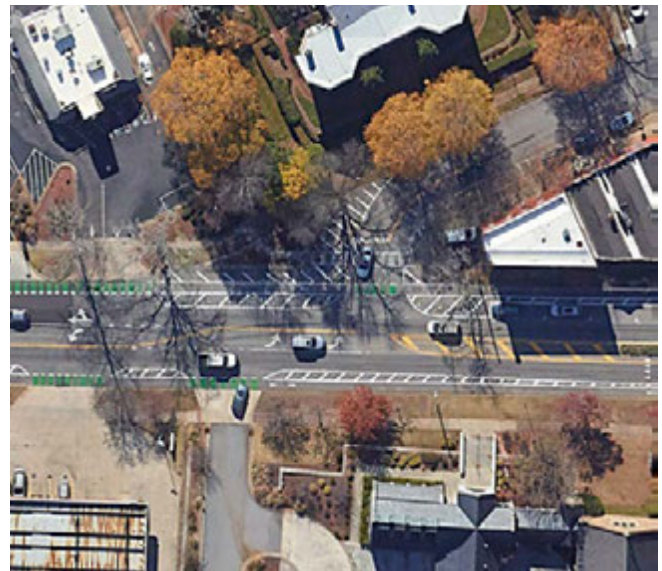
Figure 77: Improved Intersection Design After: The skewed intersection was straightened with corners that have a smaller radius, thereby reducing the speed of turning vehicles, and reducing the crossing distance for pedestrians.
