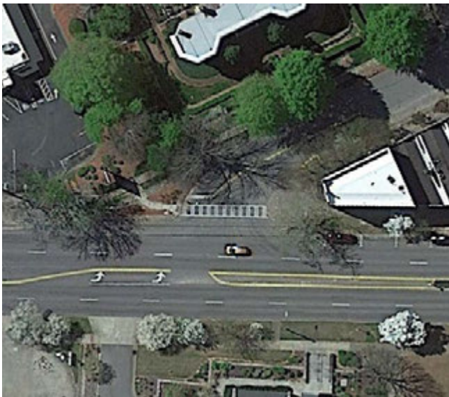
Figure 76: Skewed Intersection Issues Before: A skewed intersection with longer crossing distances for pedestrians and higher speed turning movements.
