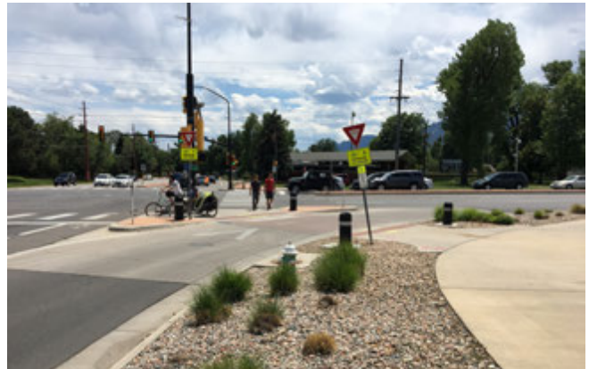
Figure 62: A well-designed slip lane should reduce vehicle speeds and provide for a safe pedestrian crossing.
