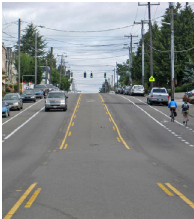
Figure 36: Two-way left-turn lanes improve traffic flow by providing a dedicated space for turning vehicles, reducing delays and enhancing safety for drivers, cyclists, and pedestrians.
