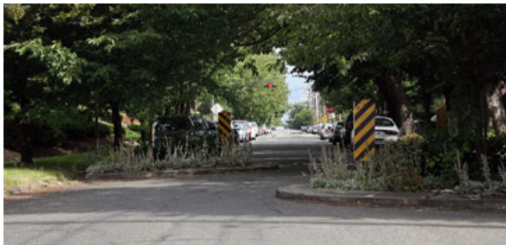
Figure 39: Chicanes are traffic-calming features that create a curved path for vehicles, encouraging slower speeds and improving safety for all road users while adding visual interest to the streetscape.
