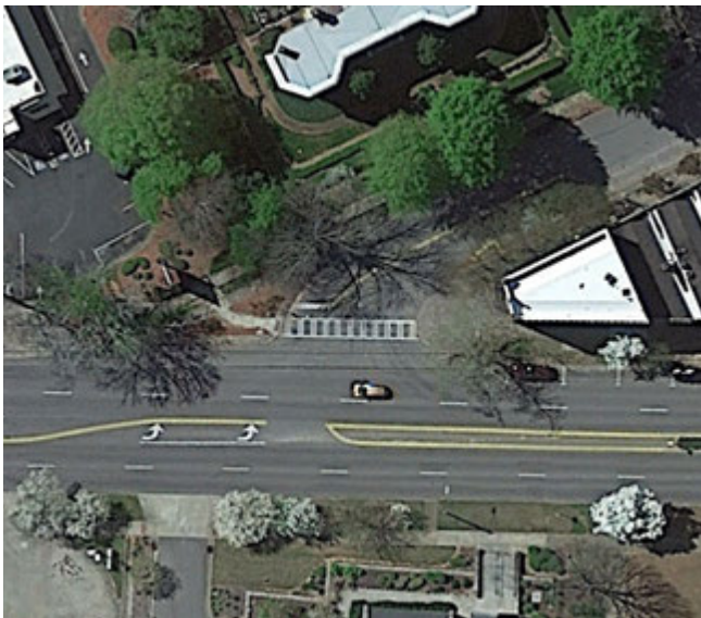
Figure 76: Before: A skewed intersection with longer crossing distances for pedestrians and higher speed turning movements
