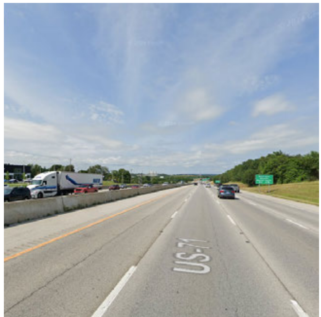
Figure 4: Primary Corridor Interstate 49, Fayetteville
