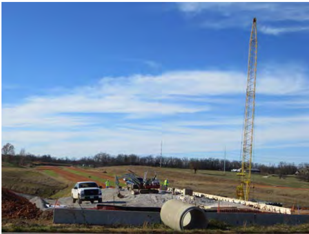
412 Northern Bypass Construction in Springdale
